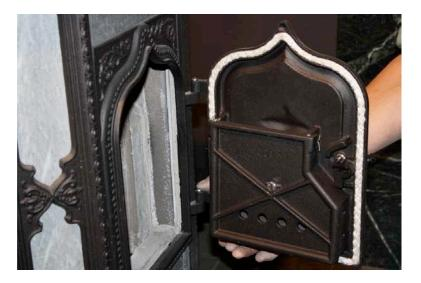
3. Lay the door face down on a suitable work surface. Use a putty knife or screwdriver to remove the old gasket. A wire brush may be used to clean out any cement residue from the gasket channel. Vacuum any leftover debris from the door and gasket channel.
