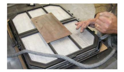
6. Allow the glue to set up for 15 minutes before placing the lid back on the stove. After waiting return the lid to the stove. Be sure the lid is properly seated on the top frame. Keep lid closed for 24 hours.
